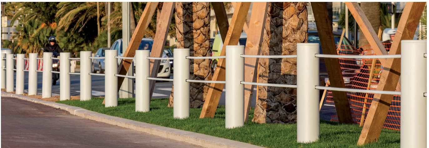
MacSafe® completed installation adjacent to pedestrian zone
