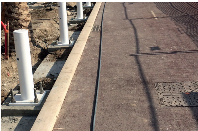
Fixing posts to ground foundations
