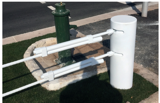
Energy absorption compression brakes
