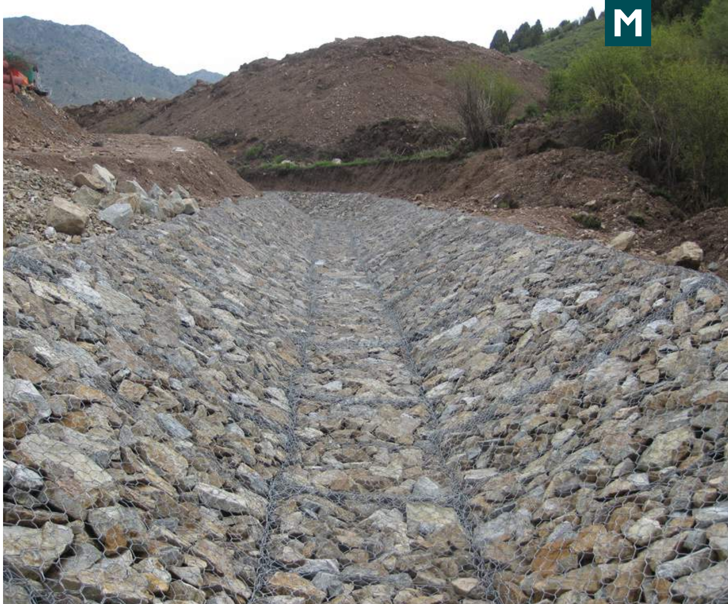
Reno Mattress lining to storm water channel, Kyrgyzstan
